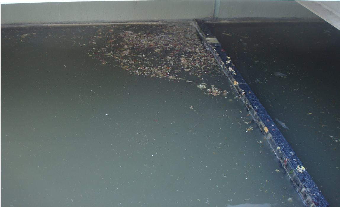
Figure 2.6 Food Waste Floating in the DWRF Primary Clarifier
